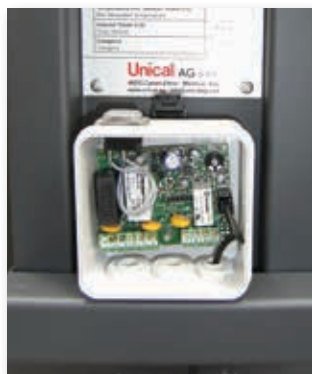
■ Temperature regulation system, with NTC sensor
